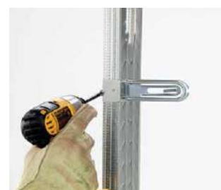
Support stays mounted to stud while securely attached with one screw
