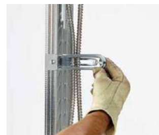
Once cables are inserted, wrap zip-tie around the end of the support to secure the cables
