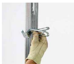
Push support onto stud
