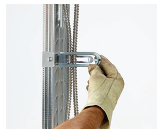
Once cables are inserted, wrap zip-tie around the end of the support to secure the cables
