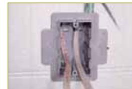
Single gang box provides 19 cubic inch capacity
