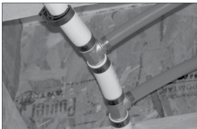
Zurn PEX large diameter tube and tee fittings shown in trunk and branch method.
