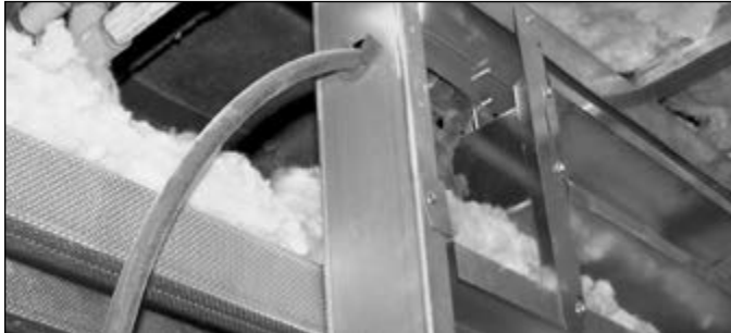
Zurn PEX tubing sleeved through steel stud for protection.
