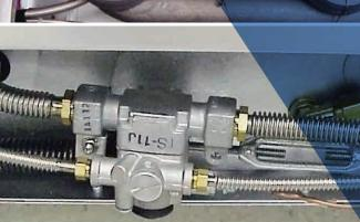
lexTube Replacement Installation Kits have been specifically designed to replace damaged internal supply lines on commercial cooking equipment. These kits are to be used as replacement components for rigid aluminum tubing. FlexTube corrugated stainless steel tubing will minimize the time spent to replace these fuel lines.
