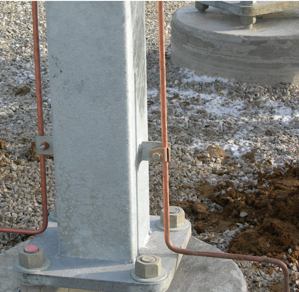
Substation earthing riser
