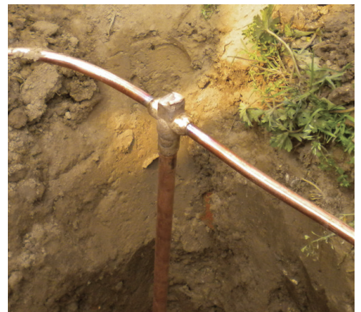
GT Cadweld connection
