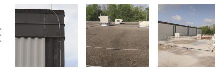
• Provides a path to ground for lightning currents
