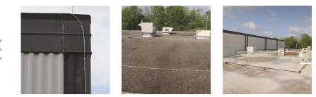
• Provides a path to ground for lightning currents
