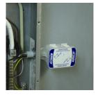
The ERICO SES40P Series of Surge Protective Devices (SPD) provide economical protection against damaging transients and surge events. These Type 1 devices are UL® Listed to UL 1449 Edition 4 and cUL® Listed to CAN/CSA C233.1. This allows installations on the line or load side (Type 1 or Type 2) of the service panel in accordance with the NEC® 2014 or CAN/CSA C233.1 without the requirement for additional circuit breakers or fuses.
