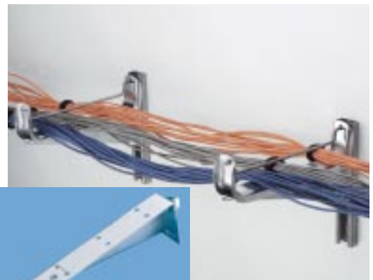
Attach U-Hook onto wall bracket already mounted on wall.
