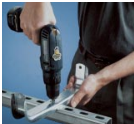
Mount U-Hook or Double J-Hook to strut.
