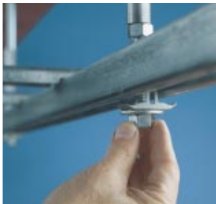
Mount strut to All-Thread Rod.
