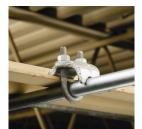
• Fix pipe or conduit perpendicular to a beam
