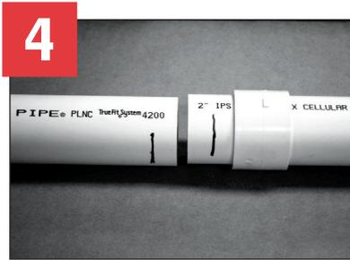
5. Apply primer between the mark and pipe end on both pipe ends.
