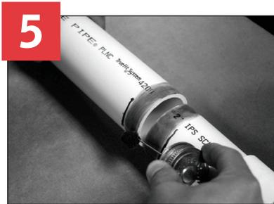
6. Apply heavy body cement between the mark and pipe end on both pipe ends.
