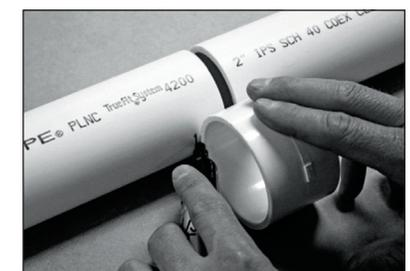
4. Place the repair coupling on the pipe with the larger pipe ID (inside diameter) end facing the gap between the pipe ends. (The larger pipe ID of the coupling has raised quarter mark lines on the outside diameter of the coupling.)
