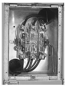
**Barriered Socket Construction** with Manual Lever Bypass
