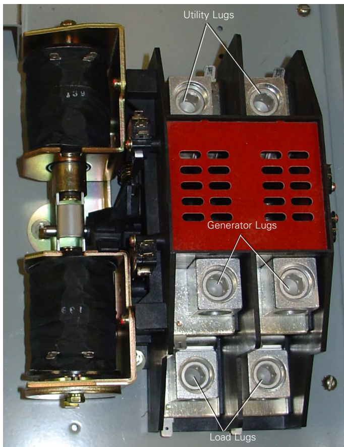
Figure 28. Replacing the 200 A Lugs.
