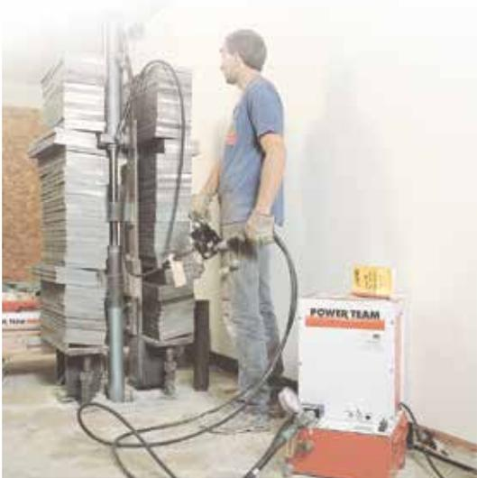
PQ- series pump used to drive piers to lift and stabilize building foundation.
