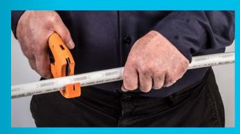
Step 1 Cut the desired length of pipe.
