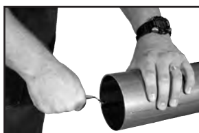
Figure 3: Deburr inside diameter deburring tool
