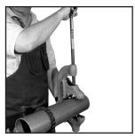
Figure 1: Cut tube to desired length using s tube cutter
