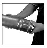
Figure 9: Inspection of final crimp
