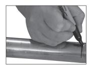
Figure 3 — Marking for Insertion Depth
