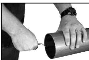
Figure 3: Deburr inside diameter deburring tool
