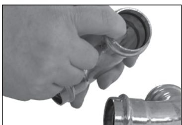
Figure 2 — Check for EPDM Seal
