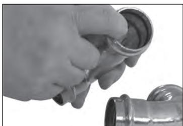
Figure 2 — Check for EPDM Seal
