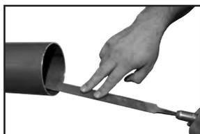
Figure 2: Deburr inside diameter using a half-round file
