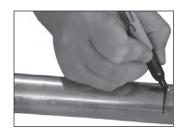
Figure 3 — Marking for Insertion Depth
