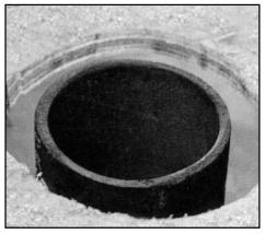
The hole in the wooden subfloor is cut too large to properly secure a closet flange.
