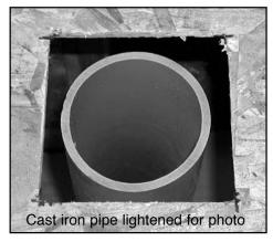
In new construction, contractors everywhere find it easier to cut square holes rather then round holes for DWV pipe and closet flanges.
