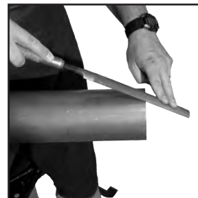
Figure 4: Deburr outside diameter using a half-round file
