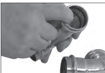
Figure 2 — Check for EPDM Seal
