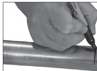
Figure 3 — Marking for Insertion Depth
