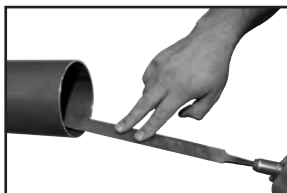
Figure 2: Deburr inside diameter using a half-round file
