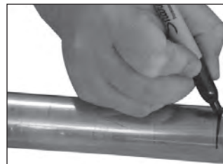
Figure 3 — Marking for Insertion Depth
