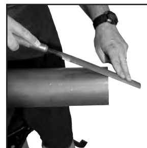
Figure 4: Deburr outside diameter using a half-round file
