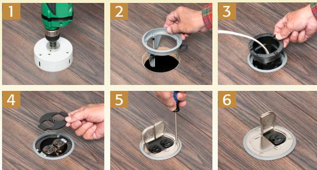
1. Determine box location, taking care to avoid structural framing members. Using hole saw cut 4-1/4" diameter opening through floor and sub floor.
