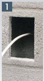
Make a 3-1/4" x 5-1/2" hole in block. Pull wiring through plastic block bushing and opening in block. Block bushing mounts to interior side of block.
