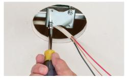
Loosen sled screws. Slide to along bracket to access the hex bar. \*\*There is no need to remove the sled.
