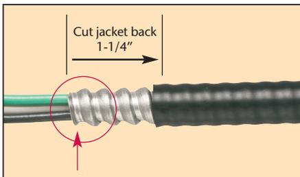
**1** Remove sharp edges from end of MC cable. Cut 1-1/4" off the PVC jacket to prepare cable for installation of fitting.
