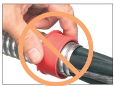
2 If you are using an end stop bushing, determine which one to use by sizing it to the cable bundle (not the metal jacket). Incorrect size shown above. The metal jacket
