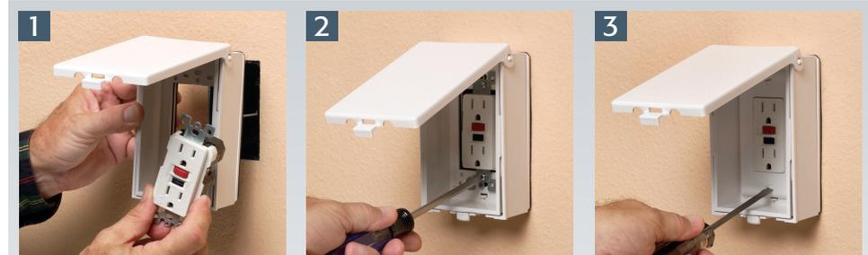
1 Feed device through opening (cover is removable for easier access).
