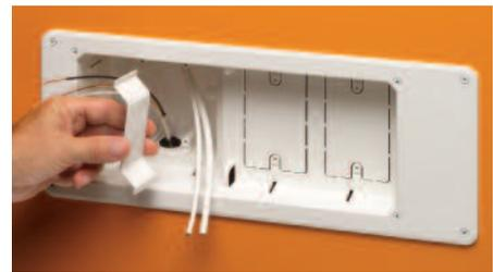
**4** Install low voltage separator if using low voltage in double-gang box.
