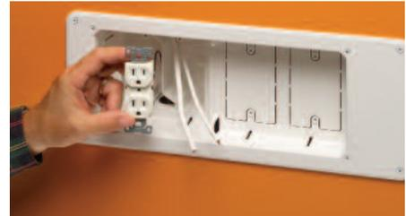
**5** Install power and low voltage wiring devices.
