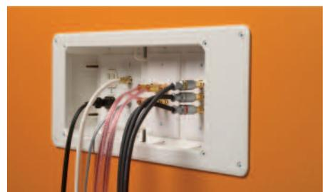
Finished installation with wires plugged in to recessed TV Box
