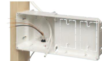
**2** Install NM cable connector. Pull power and low voltage cables.
