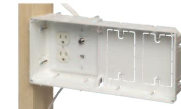
**4** Install power and low voltage wiring devices.
