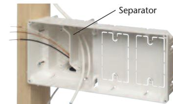
**3** Install low voltage separator if using low voltage in double-gang box.
