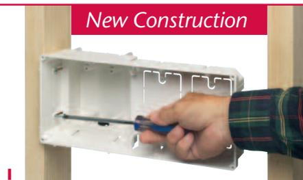
**1** Mount box section to stud through the slotted holes in box. Use minimum of (2) #6 x 1-5/8" wood screws. Positioning tabs place box properly for 1/2" finish wall thickness.
