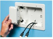
6 Attach receptacle mounting bracket to box.
