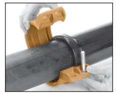
**HOUSINGS**—Place each half of the coupling housing over the gasket, making sure the housing grooved end is directed into the pipe groove.
