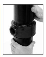
**ALIGNMENT**— Align the 5 pipe ends and pull the pipe into the gasket until the center ribs are in contact with the pipe ends. The gasket should not extend into the groove on either pipe. Rotate the gasket to align the outlet of the gasket to the same direction as the branch outlet.
