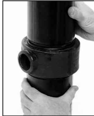
**3 ALIGNMENT**— Align the pipe ends and pull the pipe into the gasket until the center ribs are in contact with the pipe ends. The gasket should not extend into the groove on either pipe. Rotate the gasket to align the outlet of the gasket to the same direction as the branch outlet.
