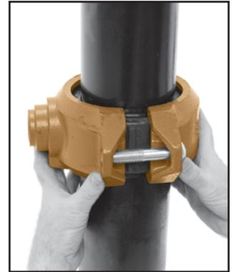
**4 HOUSING ASSEMBLY**— With one nut and bolt removed and the other loosened, place one side of the housing over the gasket. Make sure the ribs on the outside of the gasket align with the recesses in the housing and the keys in the housing are in the grooves on both pipes. Swing the other housing over the gasket and into the grooves on both sides of the pipe. Make sure the recess in the outlet of the housing is properly aligned with gasket outlet.
