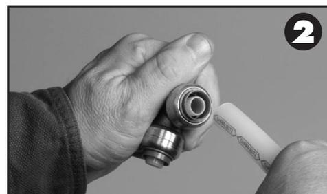
**Step 3.** Insert the tube into the fitting until the tube reaches the tube stop. Make sure the pointed end of the SharkBite pattern is even with the end of the release collar. Only when the tube reaches the tube stop has a secure joint been created.
