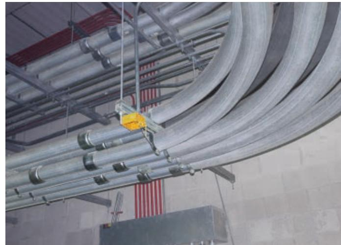
Allied's True Color EMT provides instant identification of individual power, data com, and emergency electrical systems. The 8 bright colors eliminate the need to spray, power coat or tape in the field so installation is quicker, easier and safer. All Allied EMT has the E-Z Pull™ interior finish for easier wire pulling.
