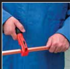
1. Using a suitable tube cutter, cut the tube end square. Ensure tube end is round and free from damage
