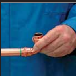
5. Using a slight turning motion, insert the tube fully up to the tube stop
