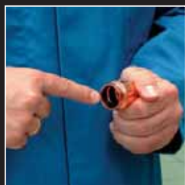
3. Ensure that the O ring is seated correctly in the fitting. Do not add oil, grease, sealants or any other additives
