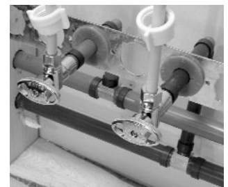
PEX Stubouts and Bracket/Grommets
