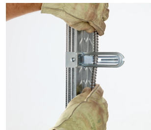
Insert cables to be secured
